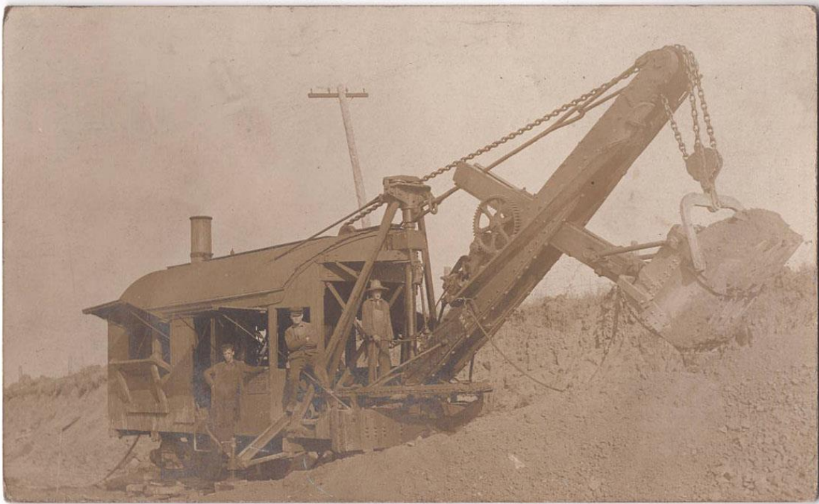
Item 614-54 – Steam shovel excavating machine RPPC – 1907, steam shovel excavating machine RPPC from Parry Sound Ont, note: a steam shovel used on the Toronto Sudbury CP Railway. To England. $100.00 SOLD
